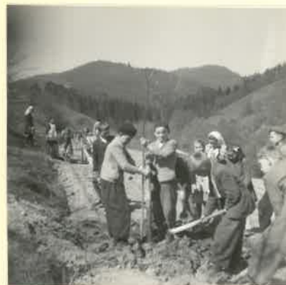
Sadenie stromkov - JRD
